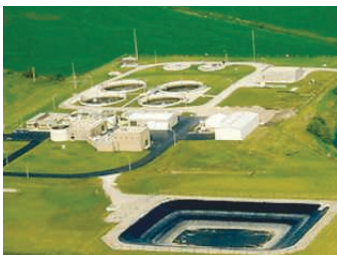
Fig. 1 CLSD with 4 Aqua SBR*1 basins ( http://clearlakesd.org/ )
