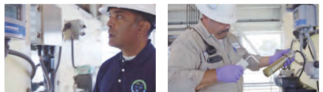
Fig 2. Ammonia meter and ion electrode maintenance.
