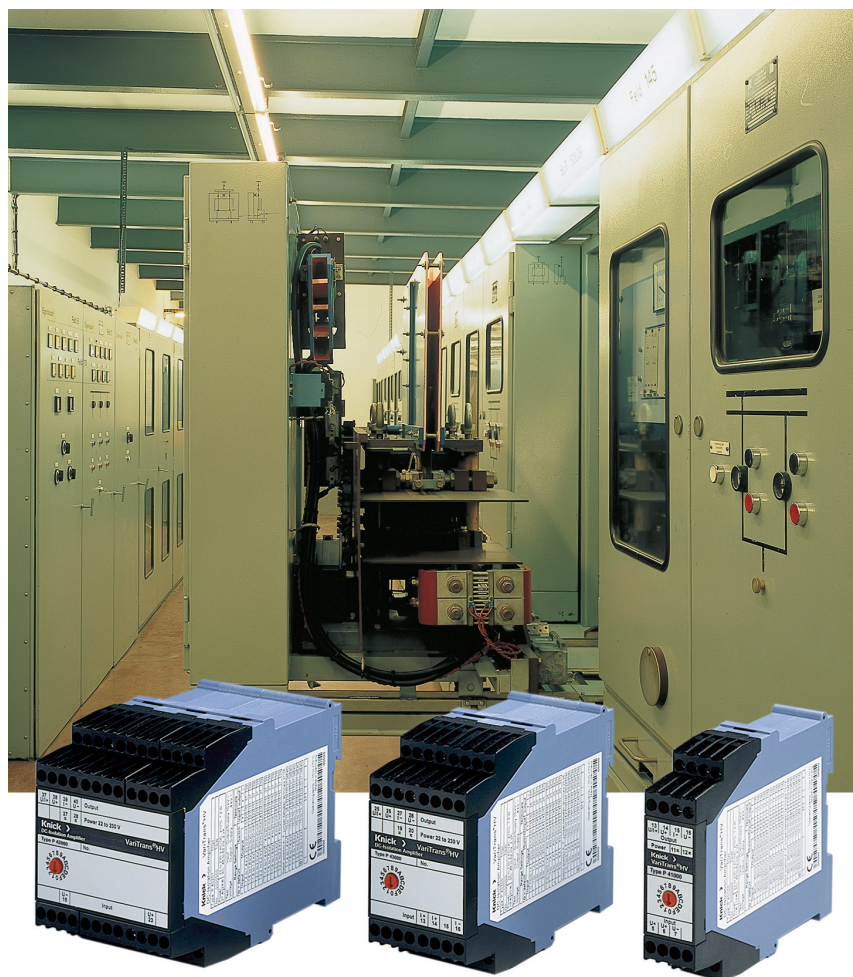
Figure 1: Switchgear for traction power supply with current and voltage measurement
