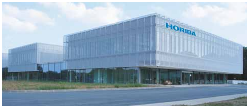
HORIBA Scientific's New R&D centre in Paris Saclay with the world's largest scientific gratings facility
