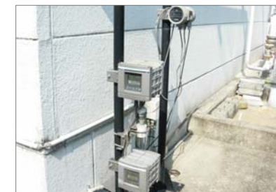
3 Providing continuous monitoring, this pH meter represents part of our comprehensive total drainage management monitoring system.
