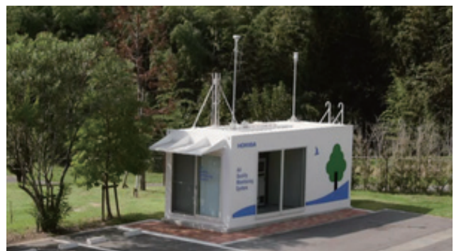
Figure 5 Air Quality Monitoring Station (AQMS)
