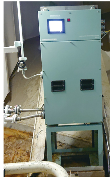
Figure 5 Installation on board
