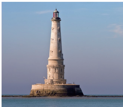
Cordouan lighthouse tenth-tallest "traditional lighthouse" in the world: 1611
