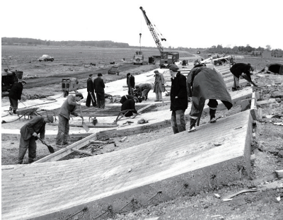
Figure 1 34° banking under construction
