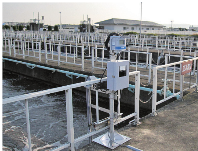
Figure 5 Field test on sewerage treatment plant
