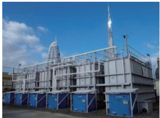
Figure 3 MBR Equipment in Burj Khalifa, Dubai
