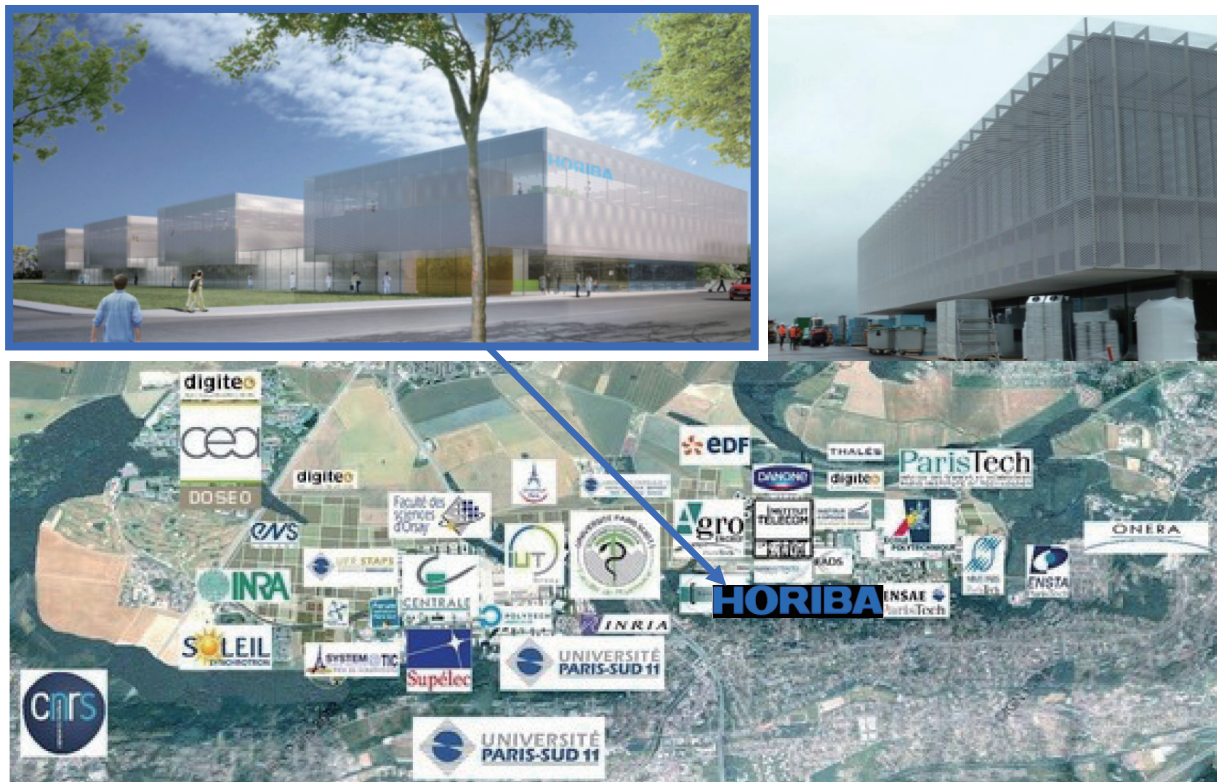
Figure 5 New HORIBA building in Palaiseau, at the heart of Paris Saclay Campus: Artist's rendering (left); building work in progress (right); Map of the research and high education places located nearby the HORIBA building on the Paris Saclay Campus
