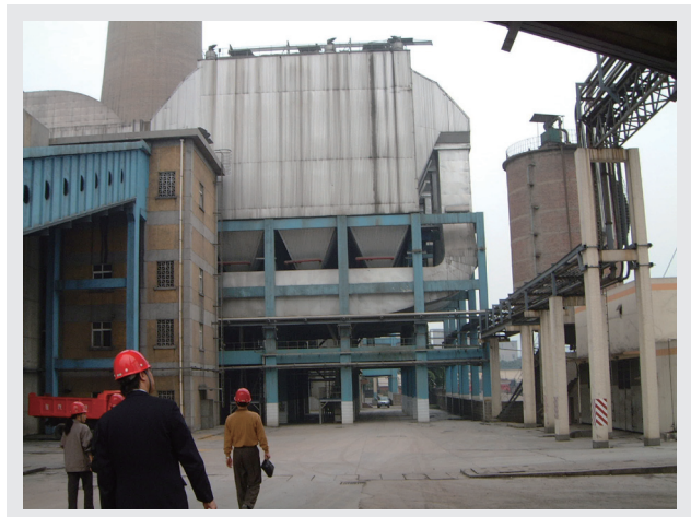
Figure 3 Electrostatic precipitator, thermal power plant
