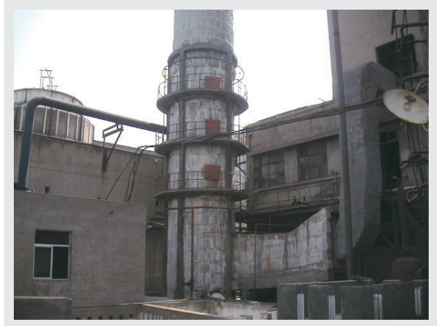
Figure 2 Desulfurization tower, general factory
