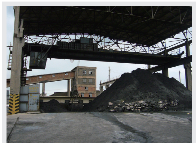
Figure 4 Coal warehouse, general factory
