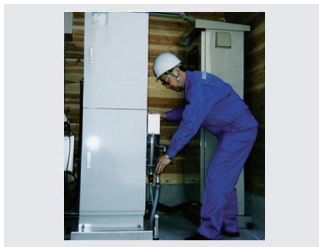
Figure 2 Installation of the TPNA-300 Automated Total Nitrogen/Total Phosphorus Analyzer
