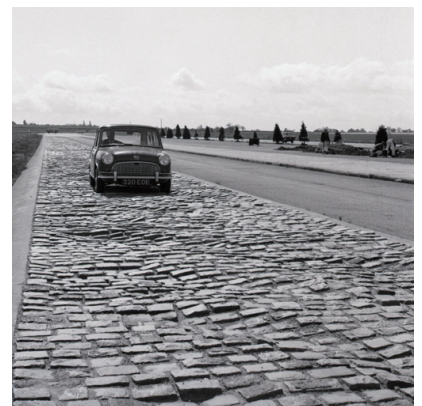
Figure 3 HORIBA MIRA's famous Belgian Pavé test facility
