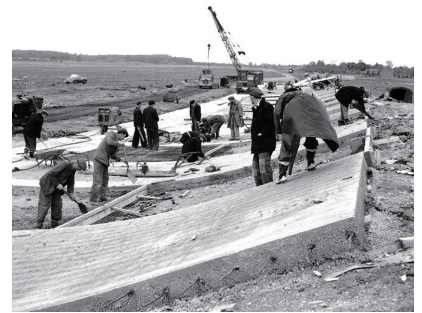
Figure 1 34° banking under construction
