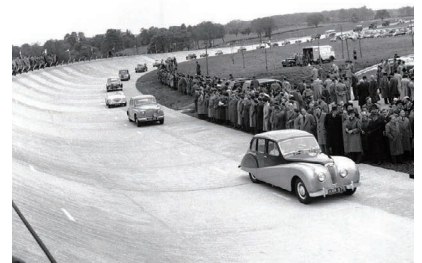
Figure 2 Opening of the High-speed Circuit
