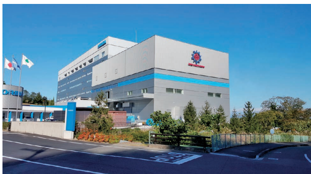
Figure 1 E-LAB(手前)とE-HARBOR本棟(奥)
