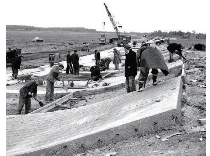
Figure 1 34° banking under construction
