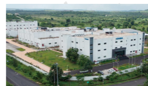
HORIBA India Private Limited, Nagpur Factory
