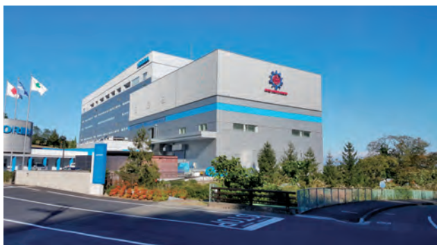
Figure 1 E-LAB(手前)とE-HARBOR本棟(奥)
